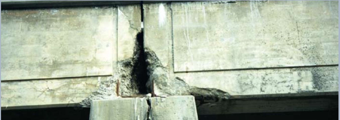
A deteriorating bridge support on a Maine bridge.
