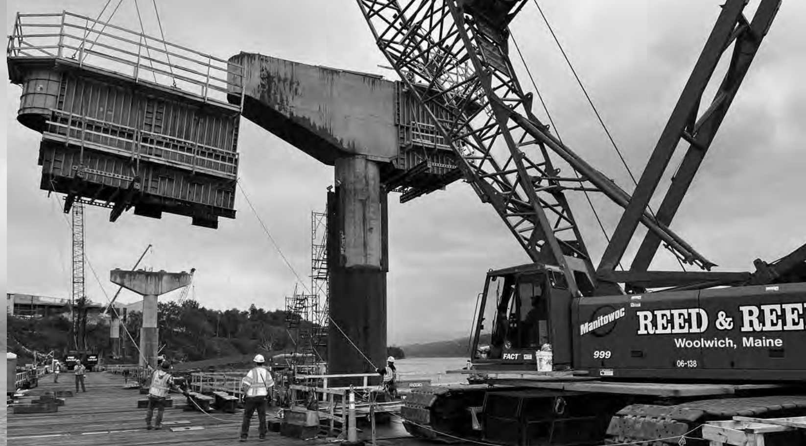
The Reed & Reed crew removes a concrete form from a recently poured bridge pier.
