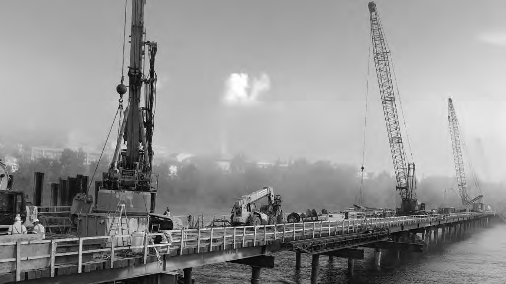
Heavy equipment on the temporary bridge that is serving as a work platform for crews from Maine and New Brunswick.
