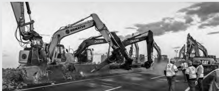
Demolition of the old Veranda Street Bridge.
