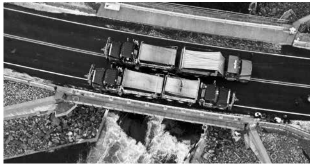
Above: The Grist Mill Bridge in Hampden was the first bridge in the nation to use FRP G beams, that are projected to be in service for 100 years. Below: Load testing a bridge, a project that has extended the working life of 100 bridges in Maine.
