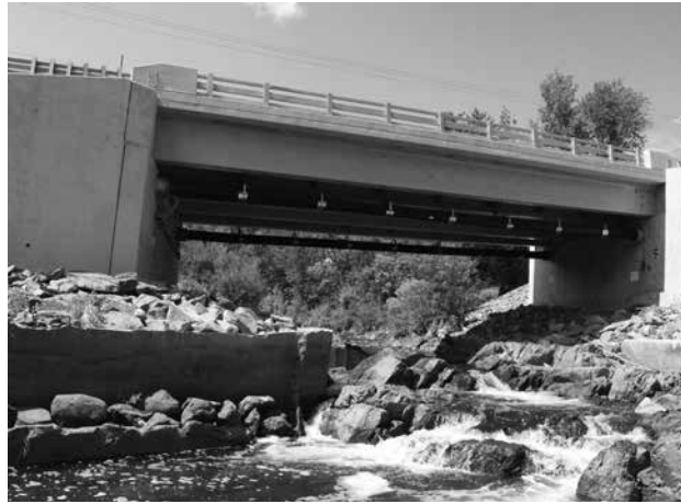
Above: The Grist Mill Bridge in Hampden was the first bridge in the nation to use FRP G beams, that are projected to be in service for 100 years. Below: Load testing a bridge, a project that has extended the working life of 100 bridges in Maine.
