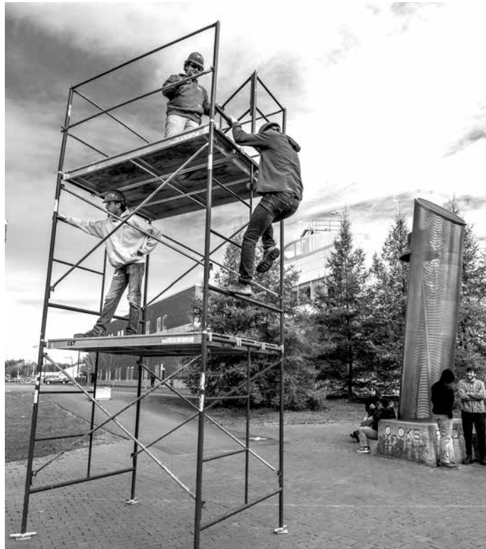
Students practice building scaffolding for a construction safety class.
