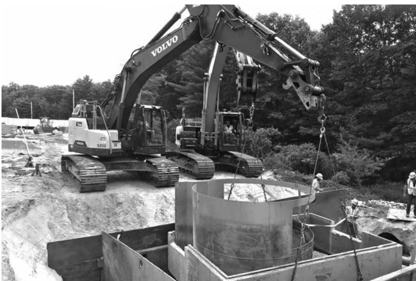
Recent projects include the Maine Turnpike Authority York Toll Plaza (top); Abbott Labs parking lot extension in Scarborough (middle); a Grondin crew sets a Vortech stormwater base in Poland Spring (bottom).
