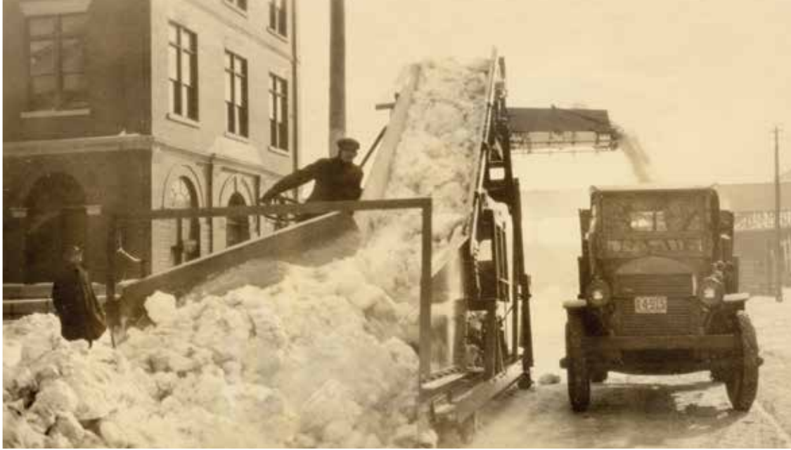
Portland Company No. 1's "Sargent" snow loader clearing snow near India Street during the winter of 1927-1928.
