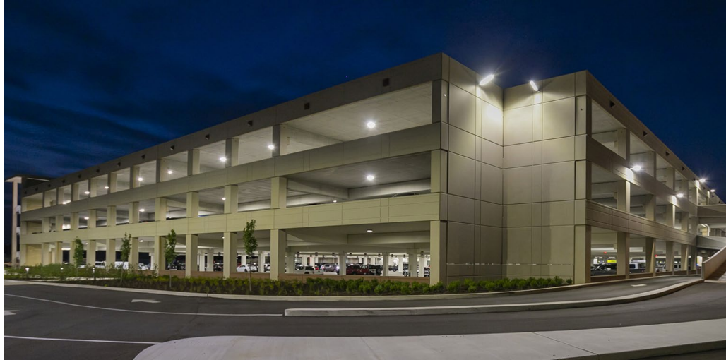
An example of an existing three story parking garage
