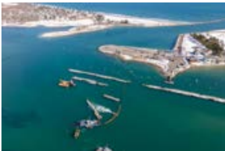
Top: York County is fortifying the coastline in Wells, while eyeing a larger $50-million project to further rebuild coastal dunes.
