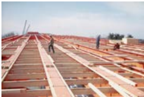
Photos: Early Piscataqua River Bridge construction in the 1970s.
