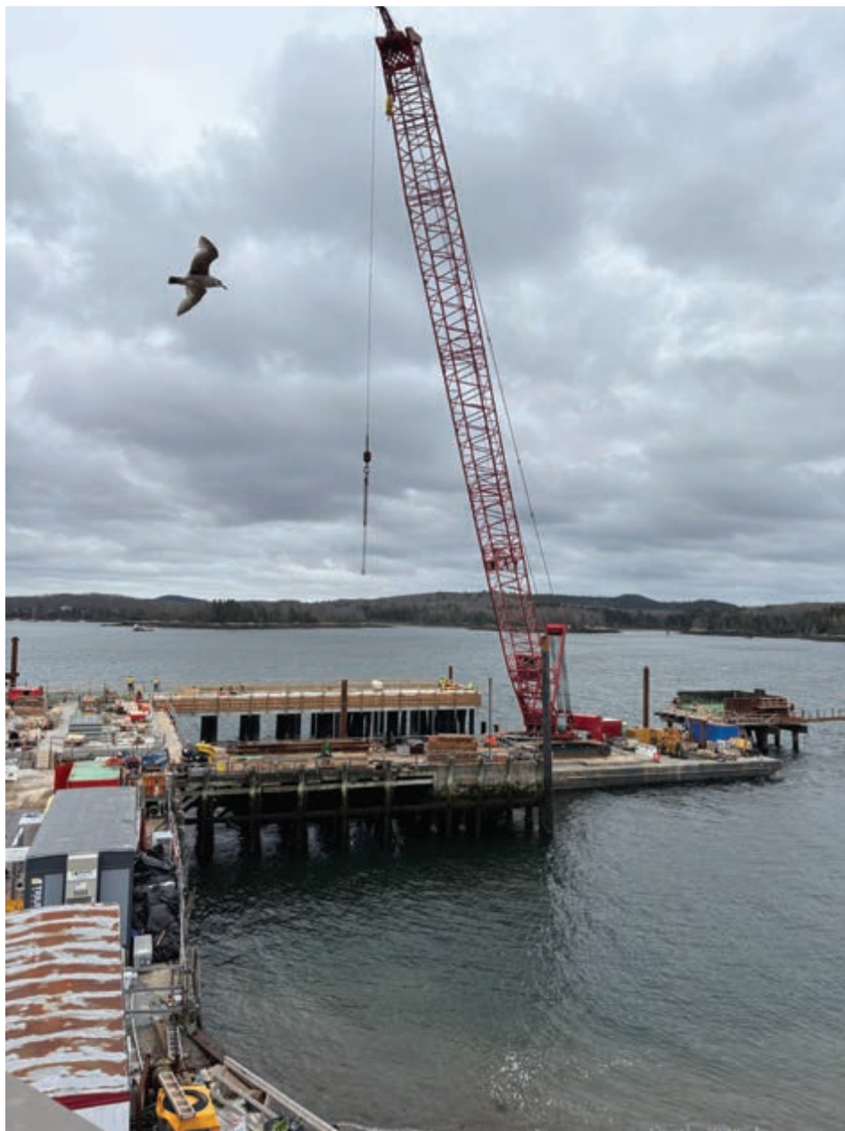
Above: Reed & Reed crane imported for the waterfront construction in Castine.
